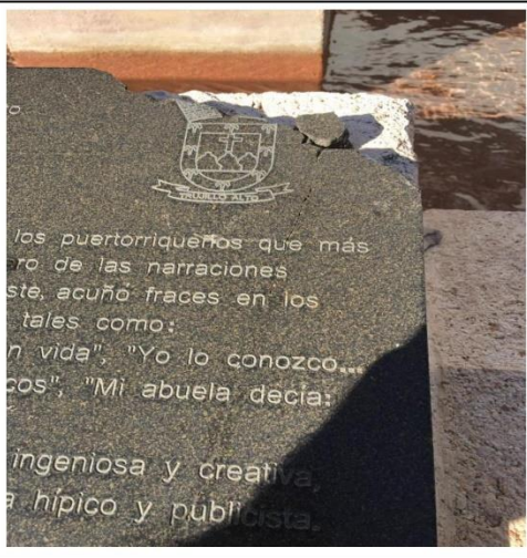
G-31 Plaza next to Coliseo; Stone plaque damage
